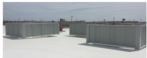
(iii.) As shown above, the screening covers multiple pieces of equipment. This is preferred over individually screening equipment, as shown below.
