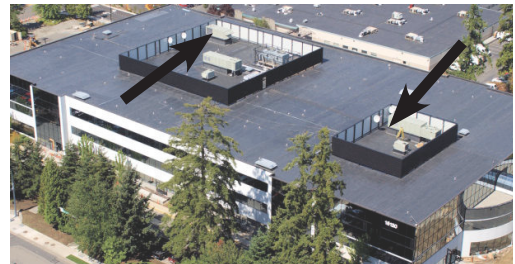
(iii.) As shown above, the screening covers multiple pieces of equipment. This is preferred over individually screening equipment, as shown below.
