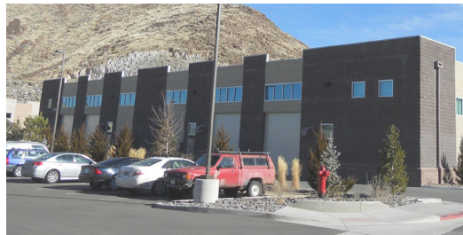
Wall recesses, height variations, material changes and repeating patterns along the entire facade.
