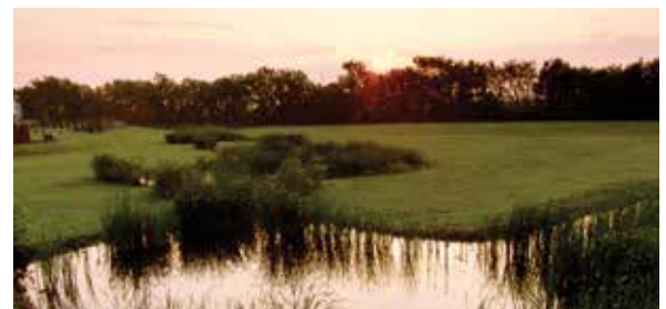
DEFORREST DETENTION BASIN
